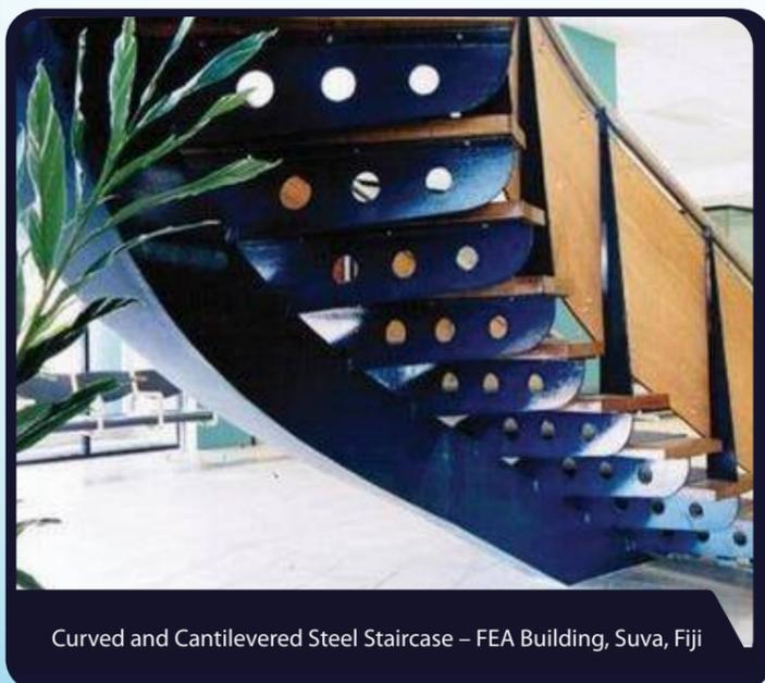
Curved and Cantilevered Steel Staircase – FEA Building, Suva, Fiji
