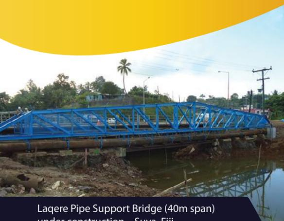
Laqere Pipe Support Bridge (40m span) under construction – Suva, Fiji
